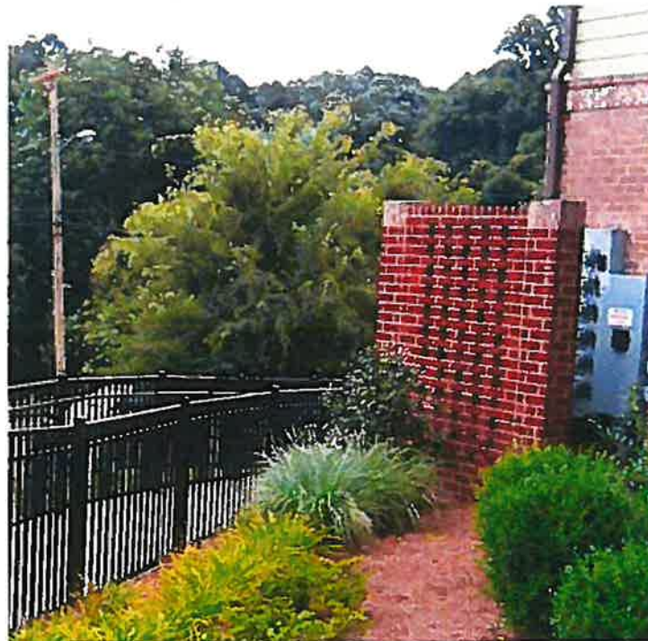
Figure 6-7-5 Service area screening
