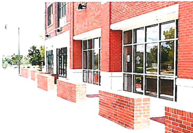
Figure 6-6-6: Facade transparency (windows) along a street facade
